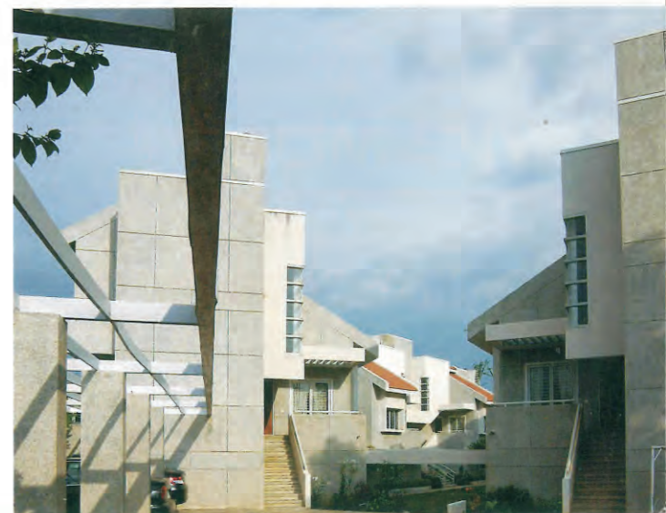
Rough finish of granite grit wash on the exterior face
